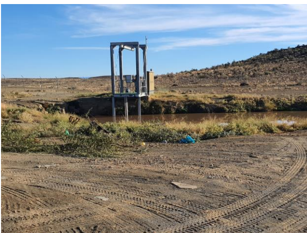
Final Storage dam
